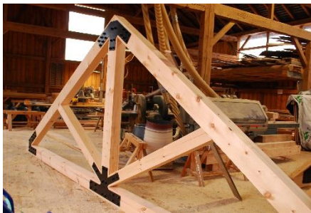
Structural Pine truss with gusset plates
